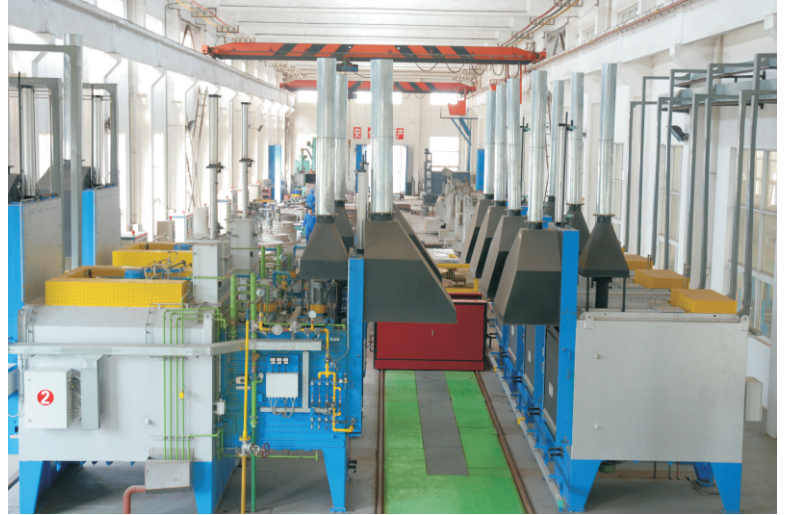
▲ Italy Ji Aifei produced heat treatment production line
